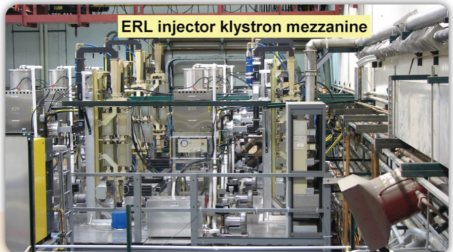
Fig. 4: Microwave generators produce the power needed to drive the superconducting linac.
