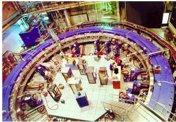
Figure 12. The storage-ring magnet. The cryostats for the inner-radius coils are clearly visible. The kickers have not yet been installed. The racks in the centre are the quadrupole pulsers, and a few of the detector stations are installed, especially the quadrant of the ring closest to the person. The magnet power supply is in the upper left, above the plane of the ring (courtesy of Brookhaven National Laboratory).
