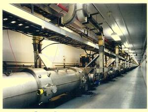
SOUTH LINAC CRYOMODULES
