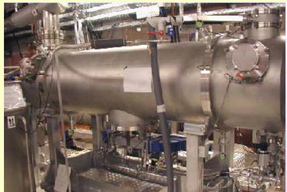
Rossendorf Cryostat, based on TESLA cavities
