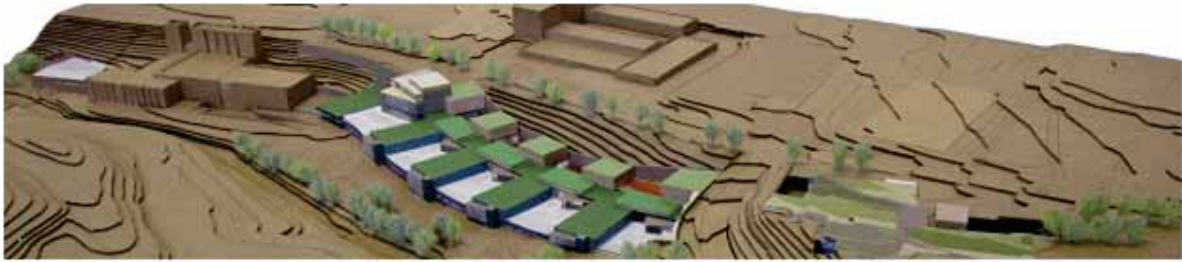
Figure 4.2.6: Model shot of aerial layout. The existing Wilson laboratory is on the left and the new experimental hall to the east of Wilson laboratory is in the center (shown with green roofs). The underground cryoplant is to the right.
