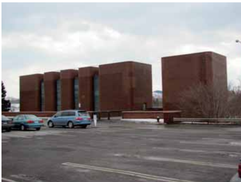
Figure 4.4.6: The Wilson Lab cooling towers.
