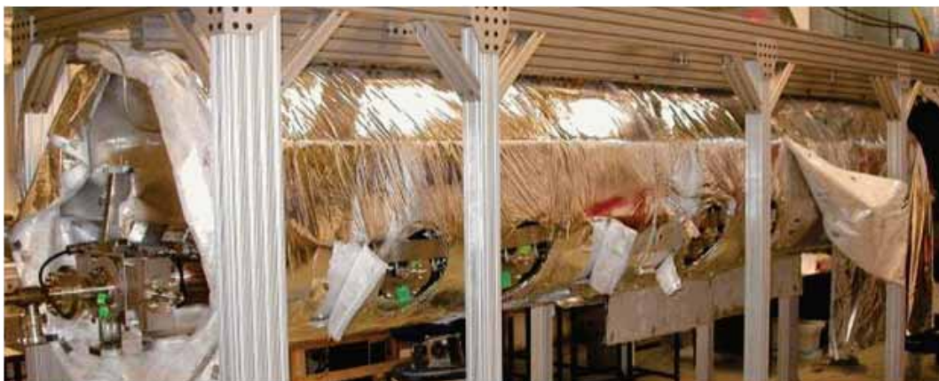
Figure 2.3.36: Photograph of the completed ERL injector prototype 100 K shield being wrapped with MLI.
