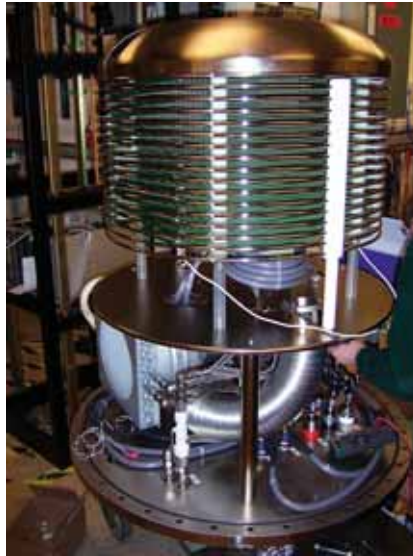
Figure 2.3.7: The HV section of the 750kV power supply. Individual circuit boards are visible inside the potential grading rings. The primary winding of the insulating core transformer is the large diameter gray-insulated wire below the circuit boards. The HV section is mounted in the pressurized SF 6 tank with its axis parallel to the axis of the gun ceramic.
