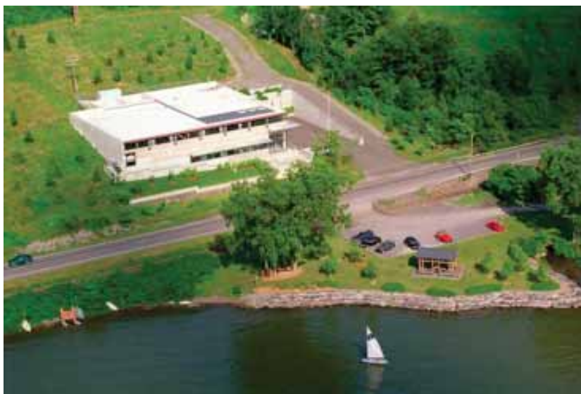
Figure 4.4.5: The Cornell Lake Source Cooling (LSC) plant.
