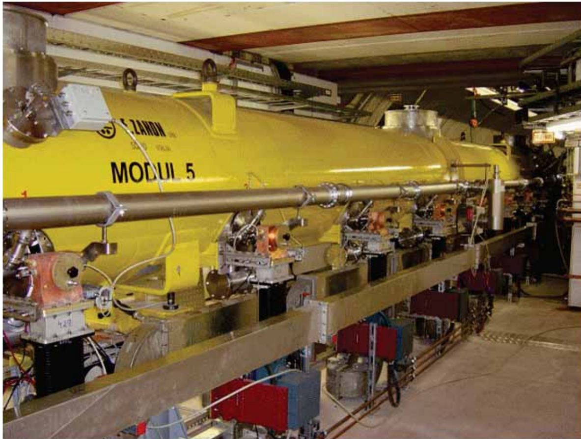
Figure 2.4.1: A photograph of a TTF-III cryomodule in the FLASH tunnel at DESY.
