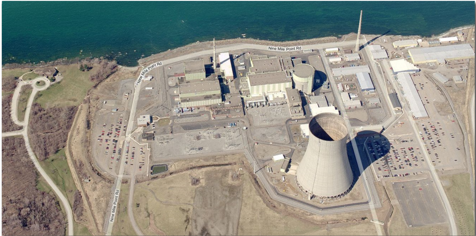
[Nine Mile Point Nuclear Power Plant, Oswego, NY]
