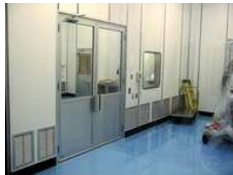
Figure 2: New 1000 sq ft clean room.
