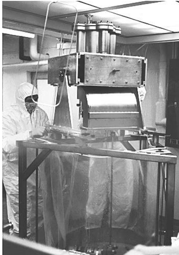
Figure: 3 BB1-2 cavity on high pressure water rinsing system.
