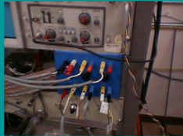
Distribution box for switches
